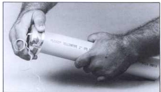
Remove any burrs from inside of pipe ends. Make sure both ends of pipe to be joined are clean, dry, and free of foreign substances. Wipe with clean, lint-free, dry rag.
