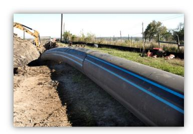
DriscoPlex® HDPE Pipe is available to meet your needs in compliance with ASTM D3035/AWWA C901 or ASTM F714/AWWA C906 and NSF/ANSI 61 product standards. Factory Mutual FM1613 product standard is also available.
